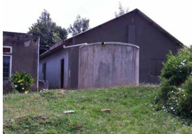
Rain water tank supplies water for 1,100 students
