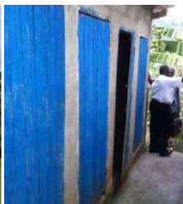
Cramped water closets
